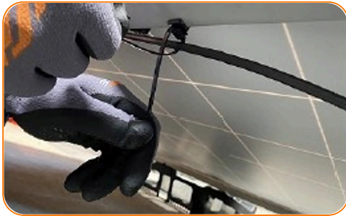
Examples of wire installation under module frame
